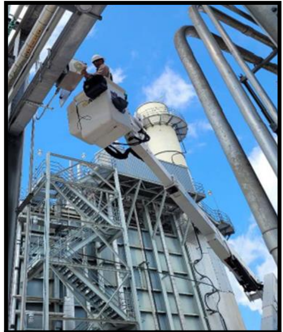
Tech installing EAS Equipment.
