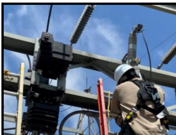
Meter Tech Installing PT/CT Units at Danevang.
