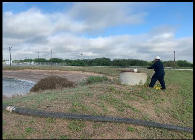
Plant personnel testing evaporation pond for leaks before the project started.
