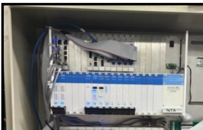
NTX-220 Retrofit Upgrade.
