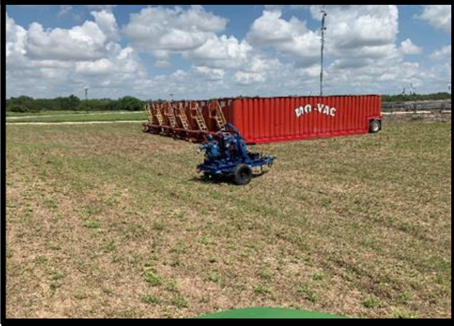
Frac tanks setup for evaporation pond water storage.
