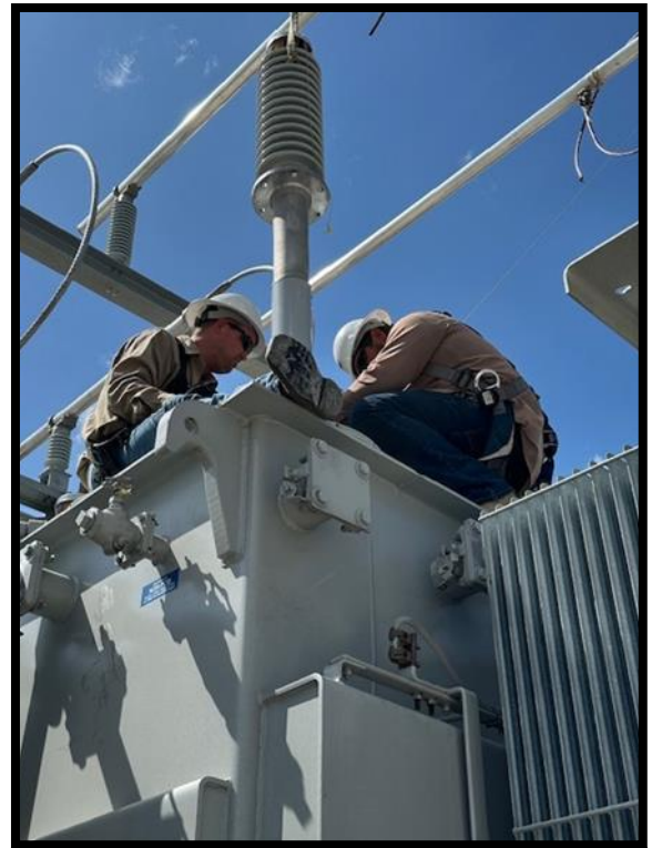
69kV bushing installation at Edna.
