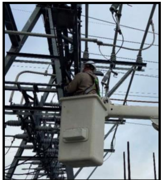
Tech removing PT at Bader.
